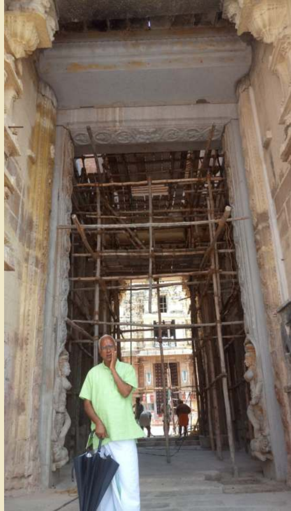
After five years of extensive renovations from 2014 to March 2019, the main RajaGopuram entrance, 10 feet width x 20 feet height was restored to its original Grandeur
