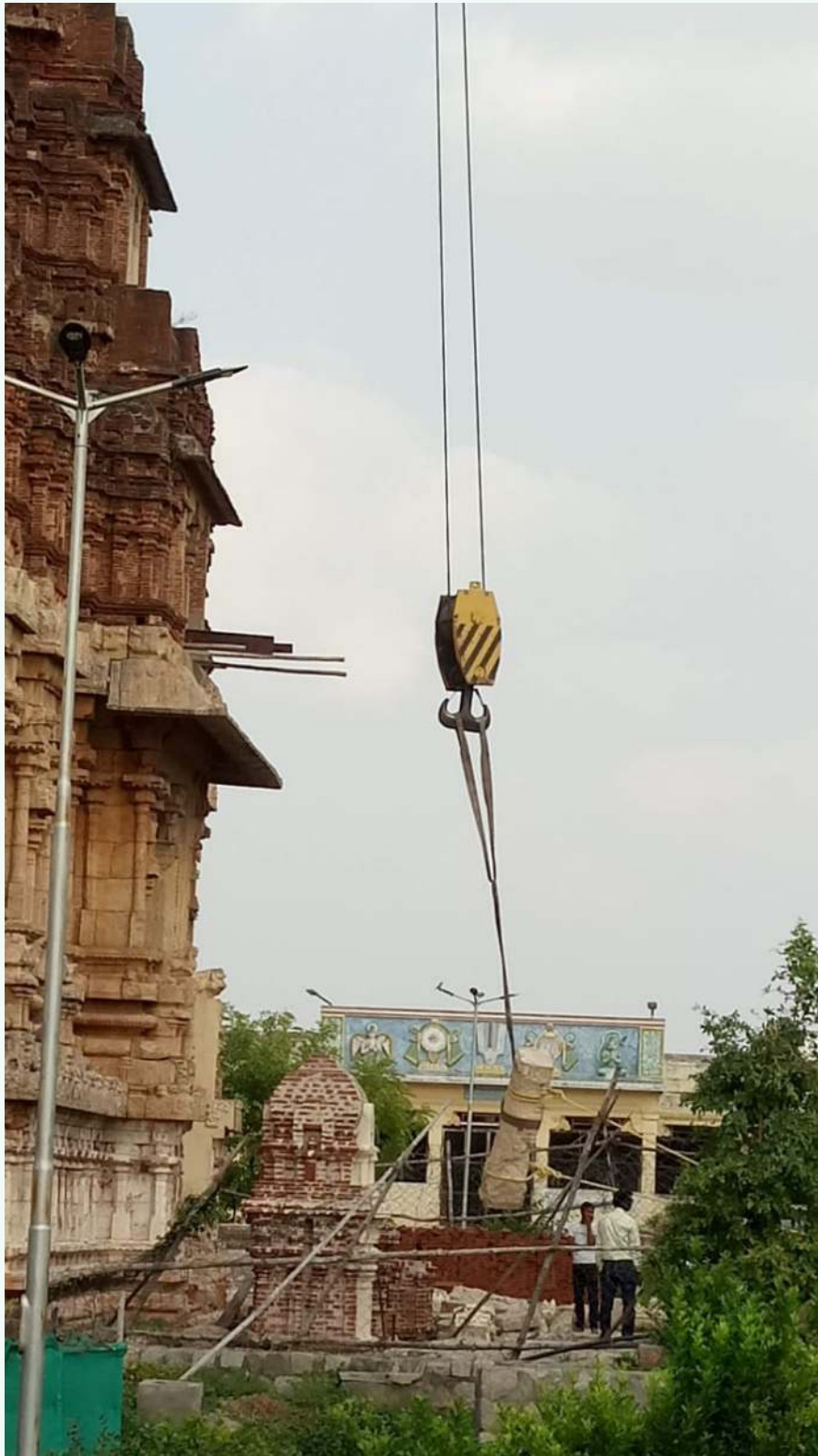
A mammoth 300 tonne crane capable of lifting 30 tons to 150 feet height was in operation handling the massive Granite pillar.
